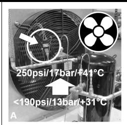
Once the operating fridge has reached a pressure of 250psi / 17bar / +41'C (in R407C-type refrigerants), the switch goes from open to closed and the fan starts running (usually via relay (for single-phase fans) or via contactor (for three-phase fans)).
